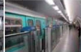
Portes palières station Invalides
